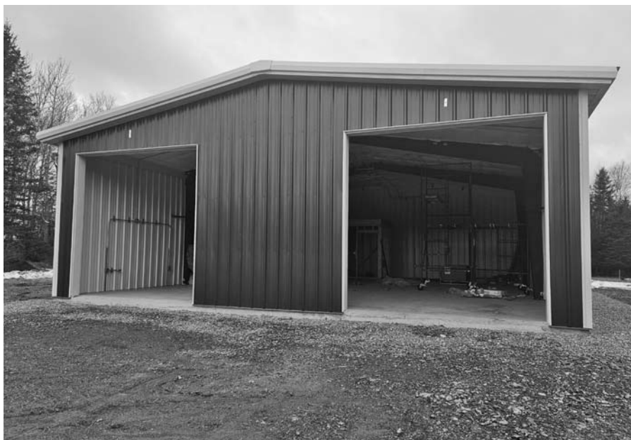
North Substation Building
