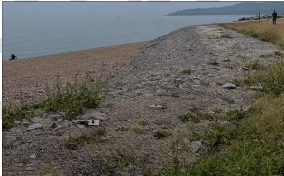
Photograph 10: Vegetation Establishing through a TECCO CELL Installation (Photograph courtesy of Geobrugg)
