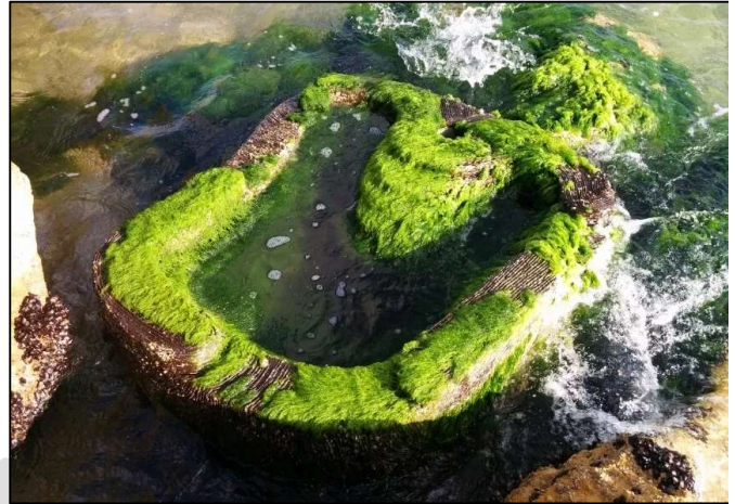
Photograph 9: Concrete "Tide Pook" supporting intertidal vegetation (Photograph Source: https://www.monmouth.edu/uci/wp-content/uploads/sites/58/2021/09/ECONcrete-Technical-Pages.pdf )
