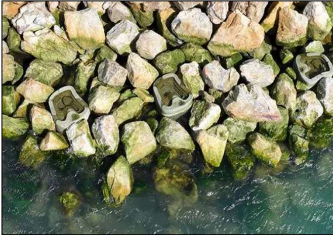
Photograph 8: Concrete "Tide Pools" integrated in a Stone Coastal Structure (Photograph Source: Nearshore habitats for marine life and coastal birds during coastal construction - EConcrete (econcretetech.com) )
