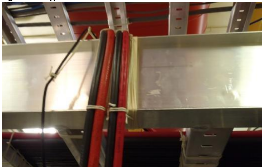
Figure 4-1: Typical Cable Transition
