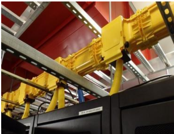
Figure 3-1: Typical Horizontal Fiber Management System
