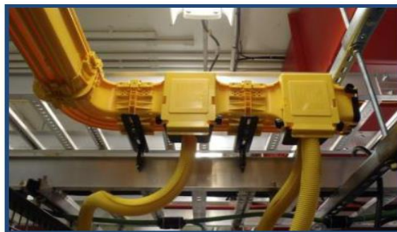
Figure 5-2: ADC Fiber System
